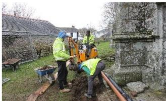
A mini digger was used to excavate the drainage channels. A perforated pipe system was installed.
