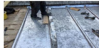
The new lead sheet is being laid in sections. Each section has to be shaped carefully despite its thickness
